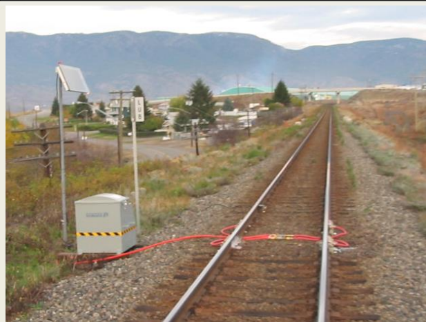
Current best practice is to apply liquid friction modifier from a trackside system
